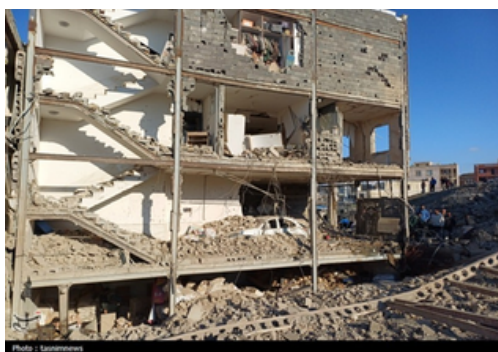
A damaged housing block in Iran (Tasnim News)
